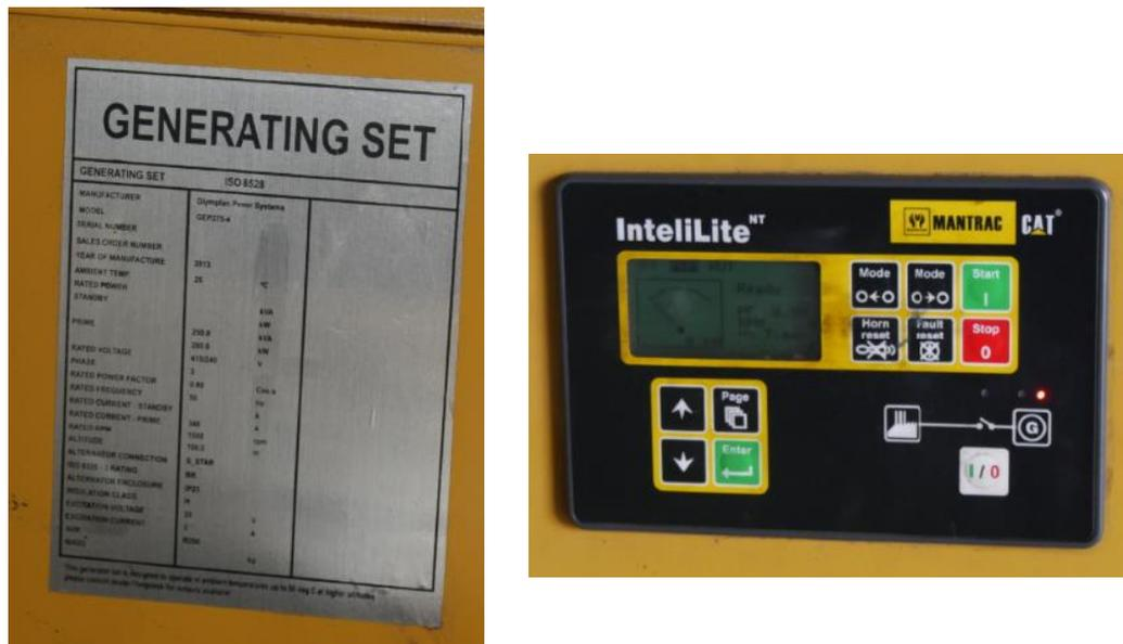
Figure 3 – Mantrac Generator nameplate and IntelliLite controller
