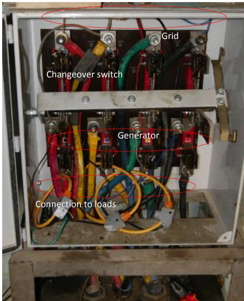
Figure 5 - Main electrical distribution panel
